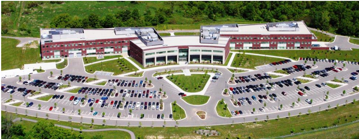
Figure 2. The ARKA Ypsilanti Township, Michigan, Facility
