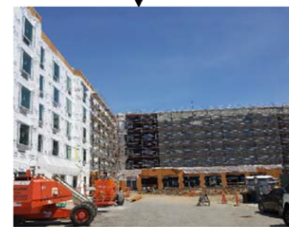
4. Siding & Roofing Outside, MEP & Finish Inside
