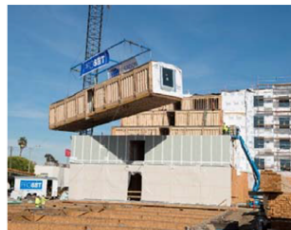
3. Craned and Connected
