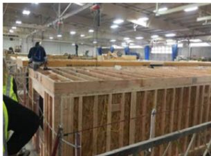
1. Modules Built in Factory
